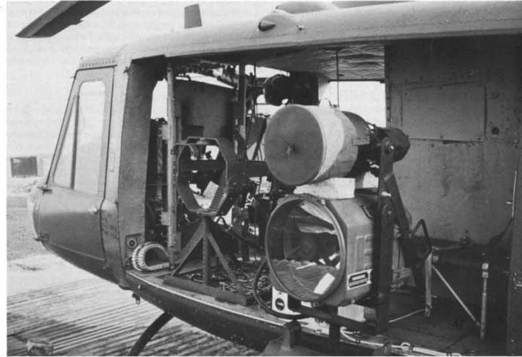
(Below) 'Killer Hawk', a Night Hawk Huey of the 187th AHC in 1970, carries a xenon light, a 'starlite' scope, and a minigun which usually had a 'stepped-down' rate of fire of 1,500 rpm. (Mike Stratton)
